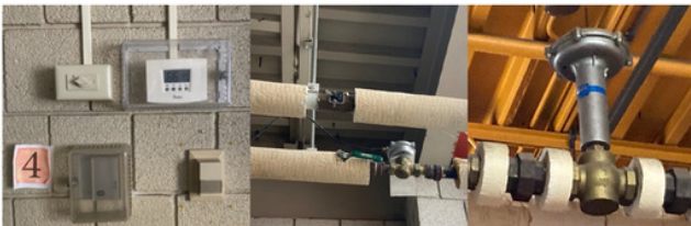
The Pneumatic Systems at LMS are 40 Years Old – 20 Years Past Their Life Expectancy
